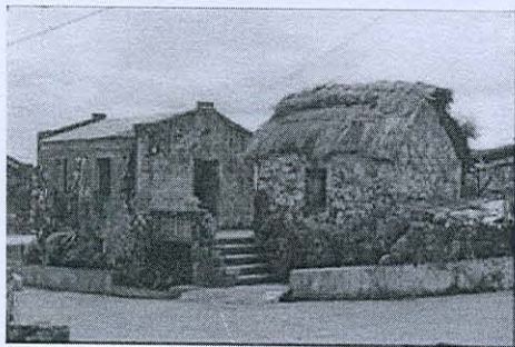
Figure 8: Houses in the Batanese Islands are built from rocks. The back wall is thick, solid and turns towards the wind. Doors and windows are but small openings and minimal in number.
